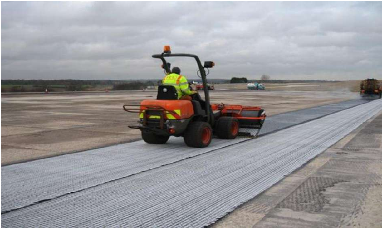
ASPHALT REINFORCEMENT (PAVED ROADS AND PAVED AREAS)
