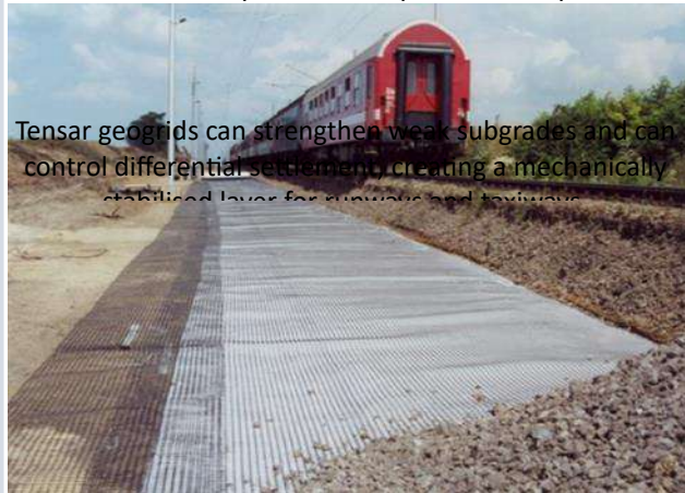
Geogrids that mechanically stabilise the track ballast layer to reduce deformation.
