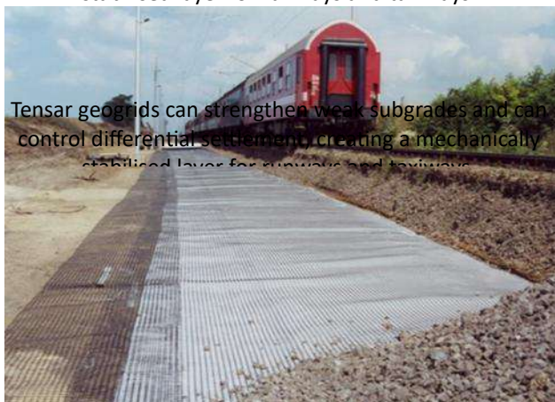
Geogrids that mechanically stabilise the track ballast layer to reduce deformation.
