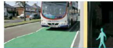
High Friction / Coloured Surfacing
