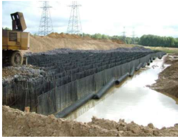
TensarTech Geocell Mattress System provides an alternative approach for embankment construction.
