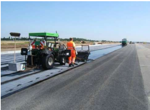
Tensar geogrids can strengthen weak subgrades and can control differential settlement, creating a mechanically stabilised layer for runways and taxiways.
